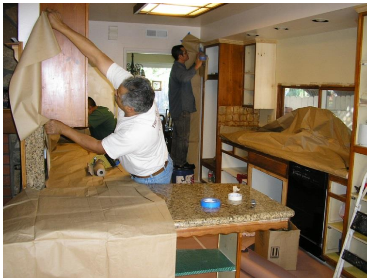
Figure 3-14. Workers Preparing Kitchen for Stripping
