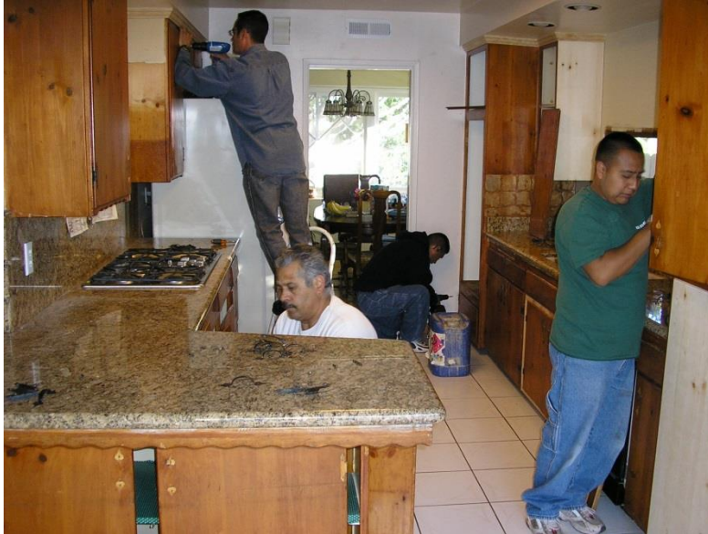
Figure 2-3. Preparing Kitchen for Stripping
