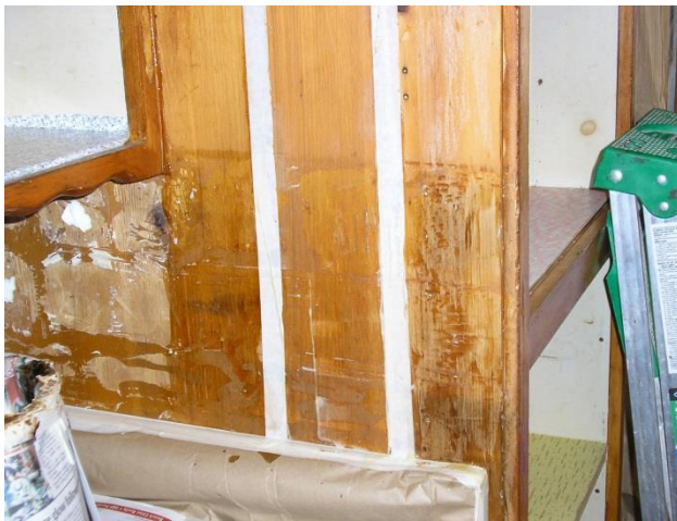
Figure 3-20. Panel #2 After Stripping
