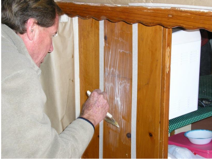
Figure 3-17. Brushing Stripper on Panel #1
